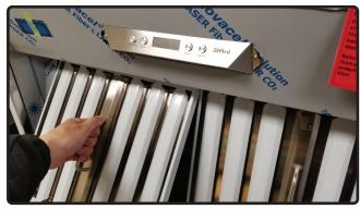
2. Remove baffle filters and duct covers from range hood.
