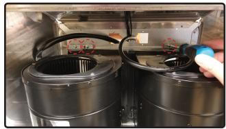
8. Position the dual blower bracket with the dual blowers into the hood body as shown. Make sure to tuck the dual blower plate into blower plate tabs. Secure the dual blower bracket by (4) screws.
