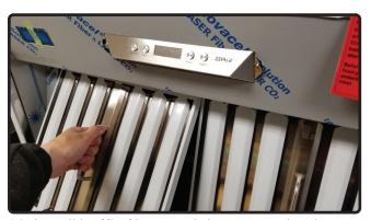
20. Install baffle filters and duct covers back onto the hood.
